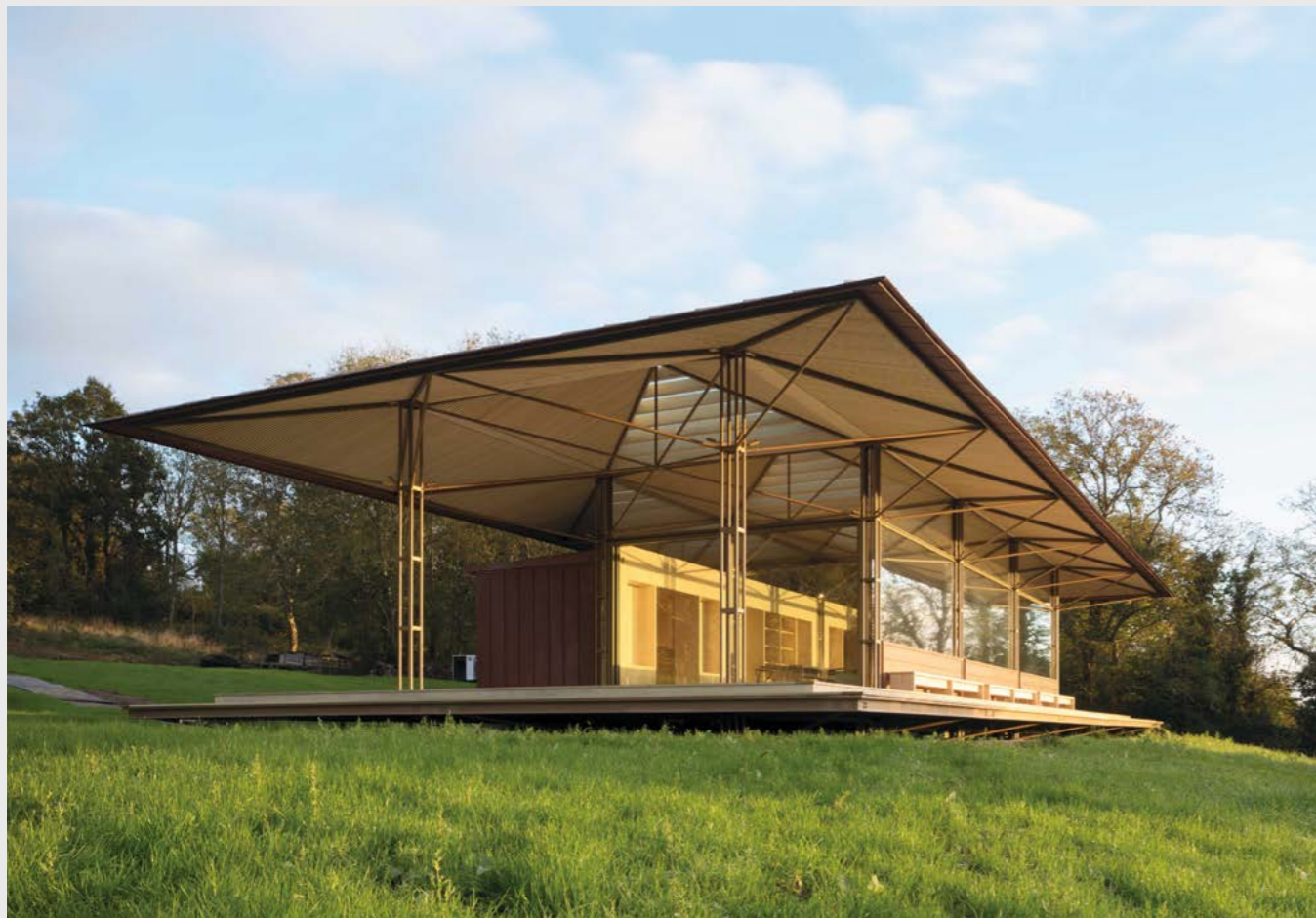
Níall McLaughlin Pavilion. Cantilevered steel and copper clad pavilion created with Níall McLaughlin Architects, Isle of Wight
