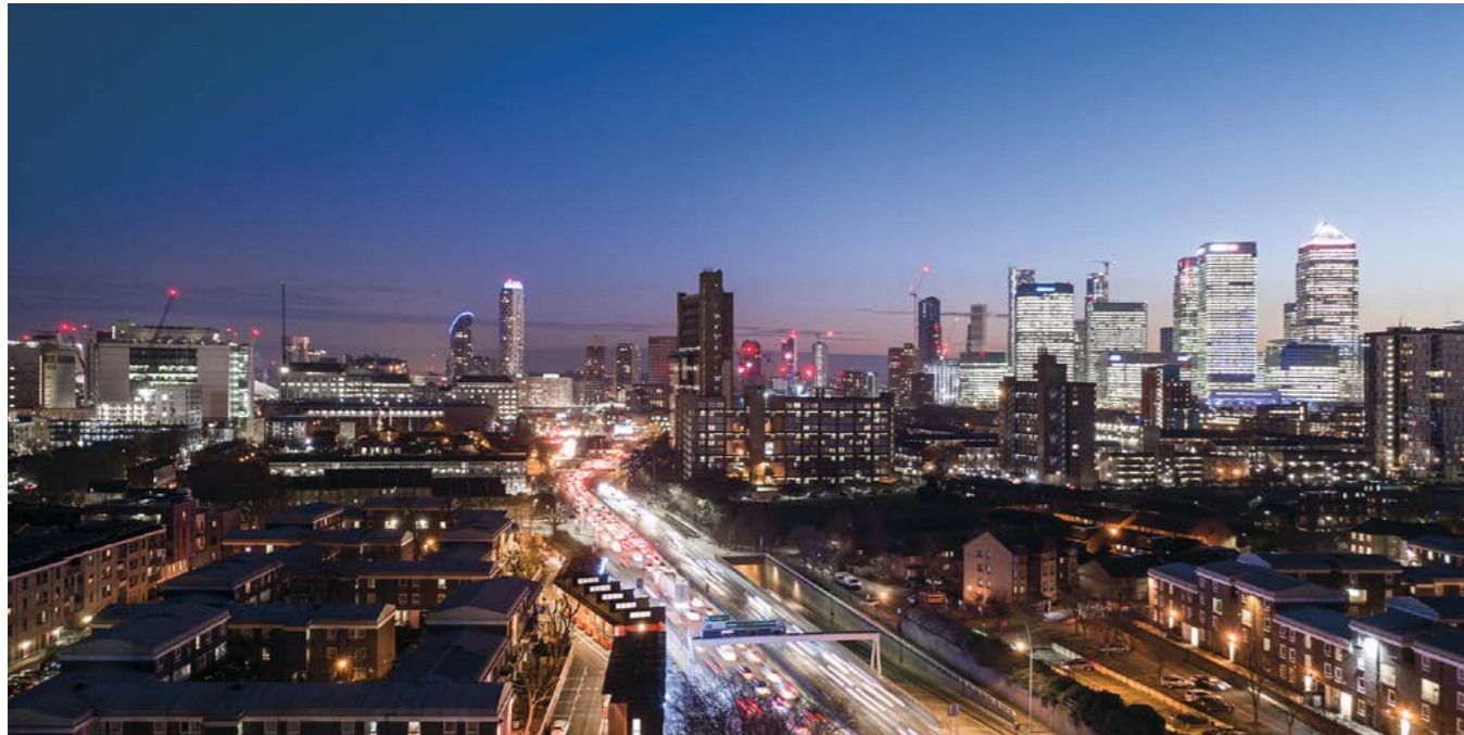
Aerial view of Poplar Works. Image – Adams & Sutherland
