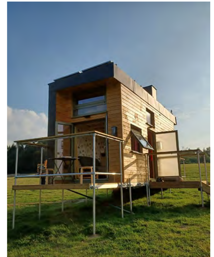
Bill Dunster's net-zero, ultra low impact flatpack dwelling prototype – achievable with small scale local production and local labour and materials
