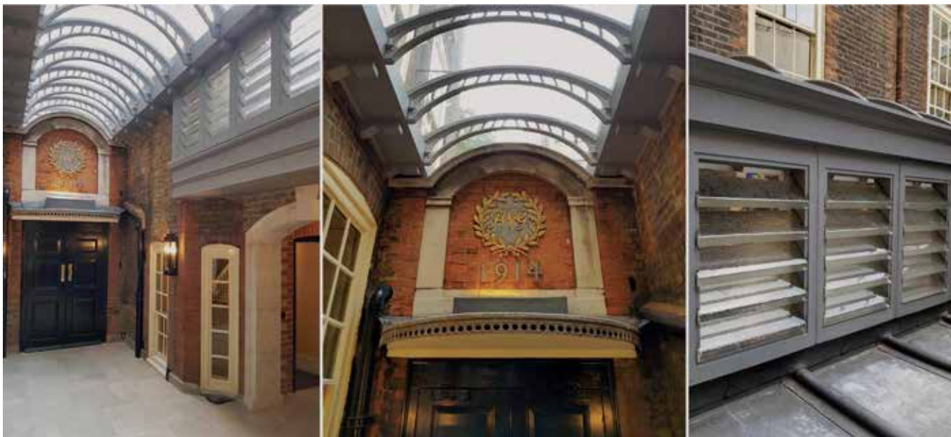
Photos of the completed roof with curved laminated glass barrel vault and fused glass louvres
